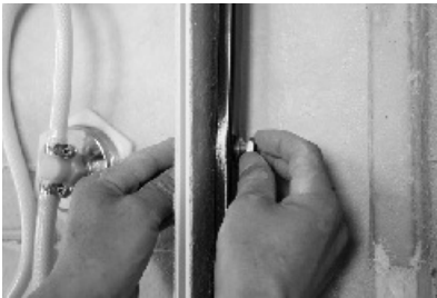
15. Put the screw into the connection hole (as picture).
