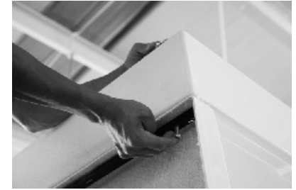
32. Set screw in the connection hole of shower body and top roof.
