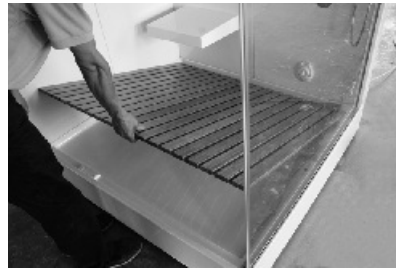
40. Install the bamboo pad.
