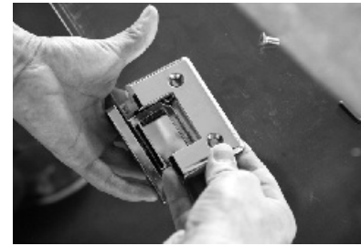
43. Fix the other hinge aiming at the hinge hole.
