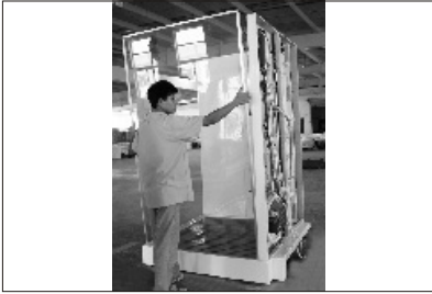
25. Install the fixed glass.
