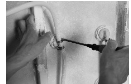
22. Screw the clip of water pipe.
