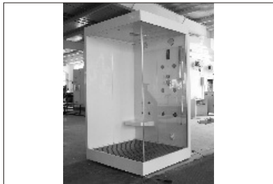
41. Check the shower body, top roof, tub tray and bamboo pad in right installation.
