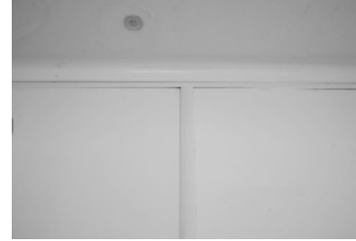
31. Fit decorative bar between top roof and back panels.
