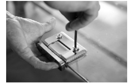
44. Screw the hinge down.
