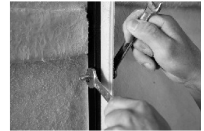
20. Screw the back panel connection.
