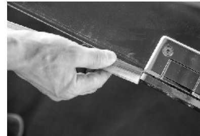
45. Install the water bar on the movable glass door.
