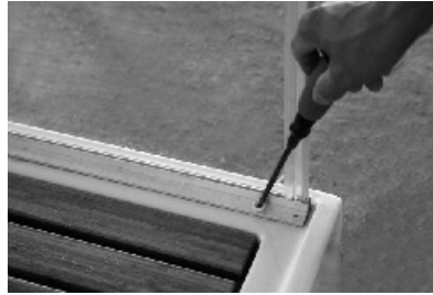
26. Screw the fixed glass to the tub tray.
