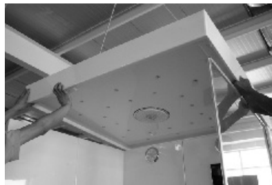
30. Put the top roof on the shower body.
