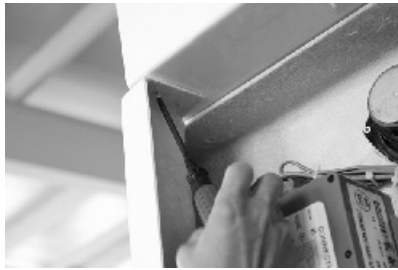
37. Screw the decorative panel to top roof.
